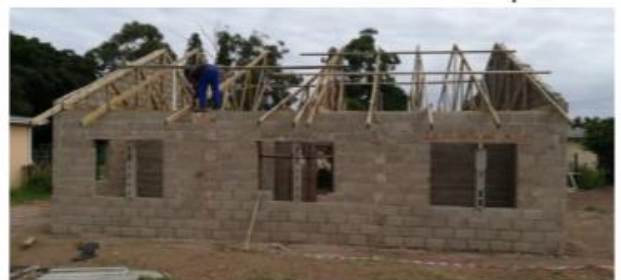
After 3 weeks the roof trusses were up:
