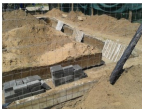
Foundations being laid
