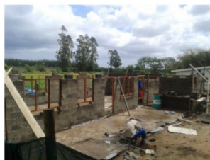
Walls are going up
